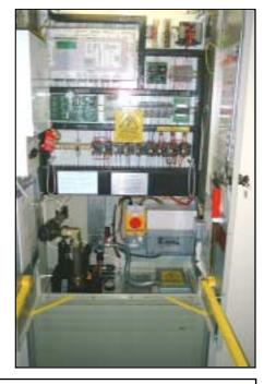
The MRC can be mounted in a recess in the shaft wall or remotely.
