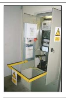
The MRC consists of a cabinet housing the control panel, 3-phase isolator and 240v consumer unit for all the lift services. The cabinet is positioned on top of a new slim GMV hydraulic tank (GL).
