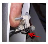
This led to a concern that the activated pit prop may not have operated the electrical switch correctly to isolate the power to the lift. In this case, it was proven that the switch worked correctly to isolate the power
