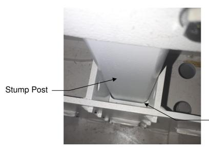
Stump post can be seen to pass through the Upper Plate (**CORRECT**)
