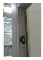
In the same way that the end spacers are countersunk and attached with extra spacers to suit so the middle spacer(s) are countersunk and attached to the frame. In addition it must be ensured that the solenoid shoot-bolt has free movement through the frame into the door lock surround.
