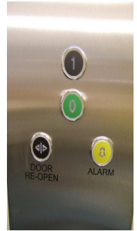
Cabin control panel
