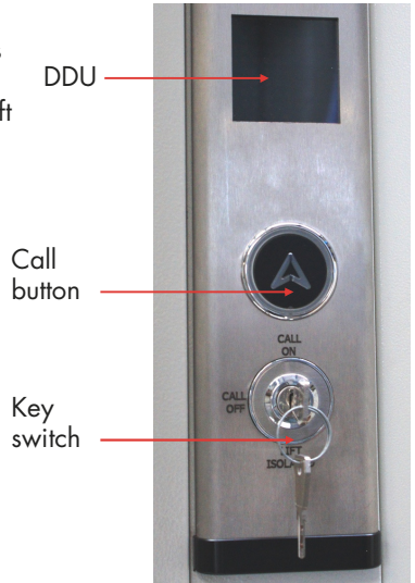
Landing control panel
