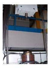
Once the ram is fully collapsed and resting on the bottom of the cylinder fit a clamp to the cylinder below the larger diameter seal housing. It may be necessary to remove the car-operating panel and fit the ram clamp through an access hole in the car panel.
